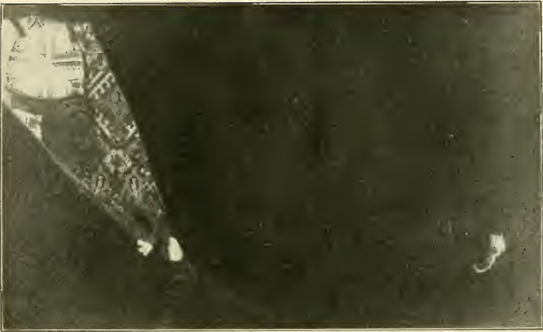
FIG. 141. AUTHOR'S FIRST FLASHLIGHT PHOTOGRAPH OF 6 MARCH, 1913. (FROM ABOVE, INSIDE CABINET.)
